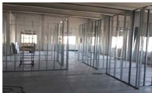
structure Cloisons Ba13 STIES
